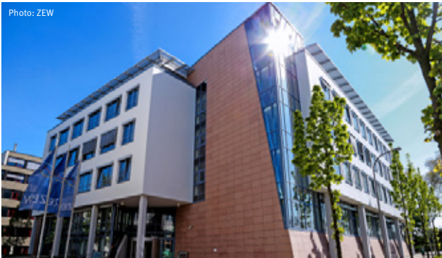
Photo: ZEW ZEW in the city of Mannheim has achieved a rating of very good to excellent as part of a regular external evaluation by the Leibniz Association.
