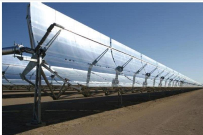
Figure 2.6: Parabolic trough concentrator
